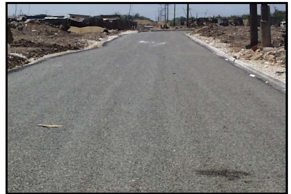
Newly constructed access road
