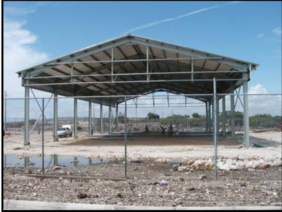
Construction of an Operations and Maintenance
