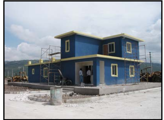
Construction of an Administration Building
